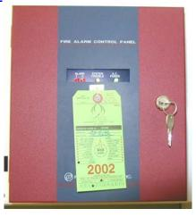
Figure 26: Fire Alarm Control Panel
