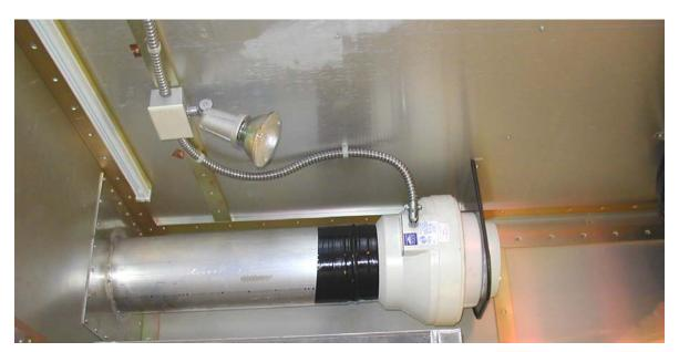
Figure 14: Magnet Room Helium Gas Exhaust Fan
