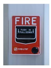
Figure 27: Fire Alarm Pull Station
