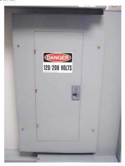
Figure 33: 120/208V AC Electrical Panel
