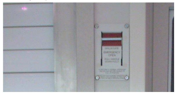
Figure 31: Roll Door Emergency Release
