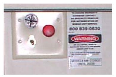
Figure 45: A/C / Chiller Alarm Panel
