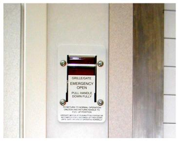
Figure 31: Roll Door Emergency Release
