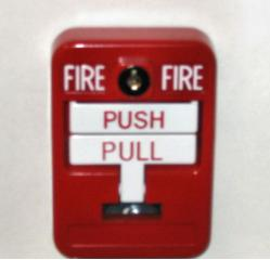
Figure 27: Fire Alarm Pull Station
