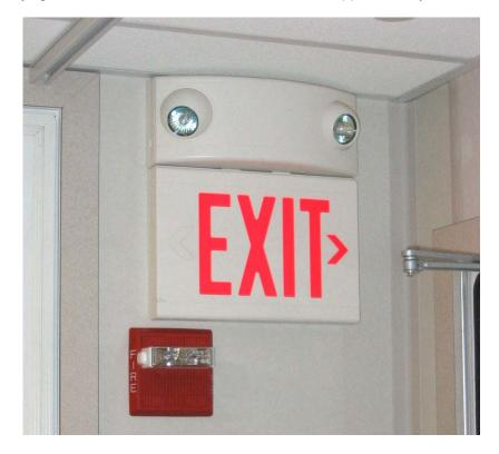
Figure 51: Emergency Dual Beam Lighting
