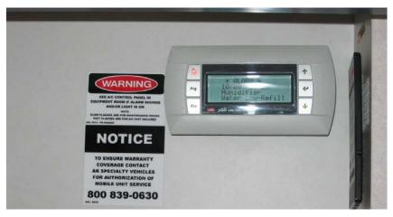
Figure 41: A/C / Chiller Alarm Panel
