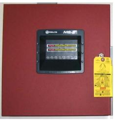
Figure 26: Fire Alarm Control Panel
