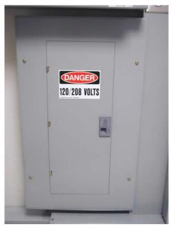
Figure 33: 120/208V AC Electrical Panel
