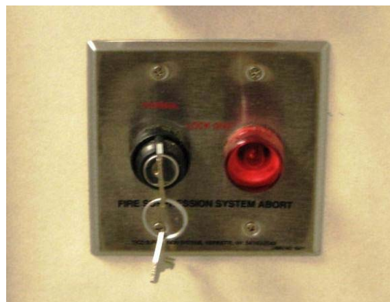
Figure 22: Maintenance Switch
