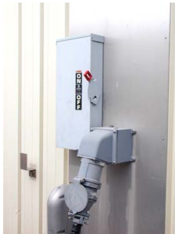
Figure 28: Shore Power Connection
