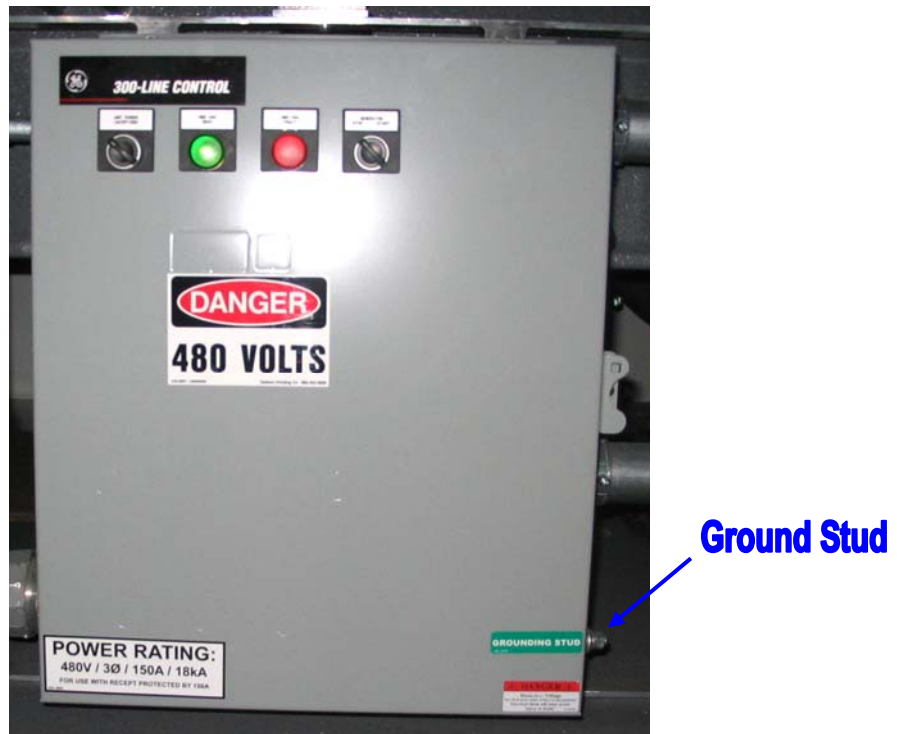
Figure 29: Ground Connection
