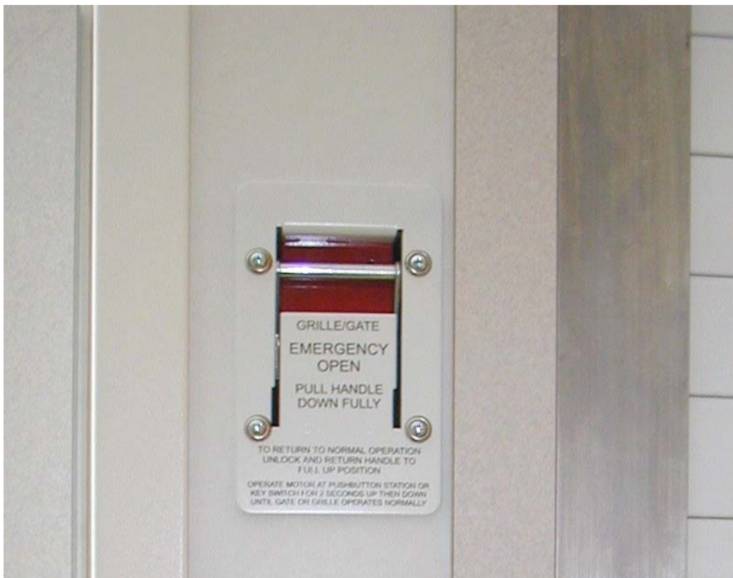
Figure 24: Roll Door Emergency Release
