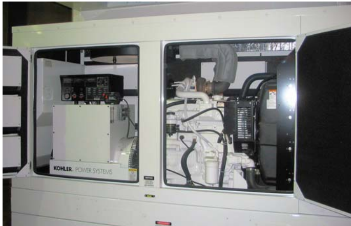
Figure 32: Generator Compartment
