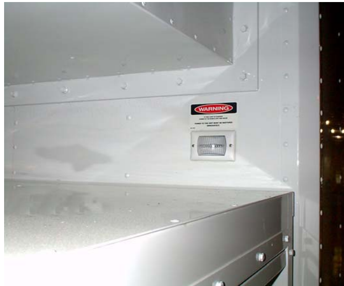
Figure 52: AC Power Loss Light
