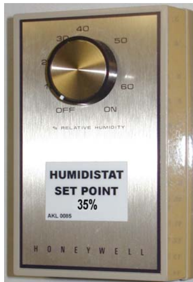
Figure 34: Humidity Controller
