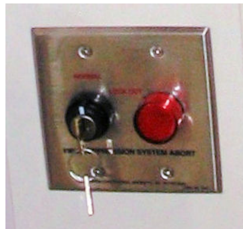
Figure 23: Maintenance Switch
